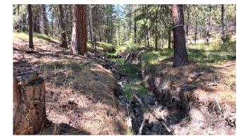
Incised section of Dick Creek currently undergoing channel fill and large wood placement, as part of Upper Trout Creek Tributary Rehab project with FS partners. Incised channel is being filled with natural materials borrowed from adjacent decommissioned road.
