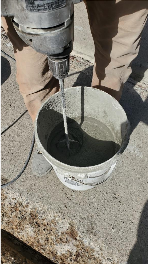
Mixing and pouring grout between bridge stringers – August 30, 2023
