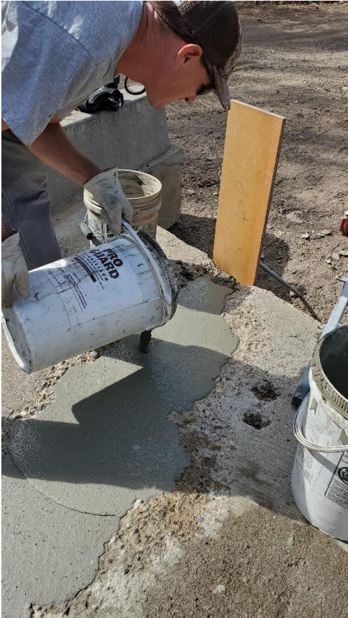
Mixing and pouring grout between bridge stringers – August 30, 2023
