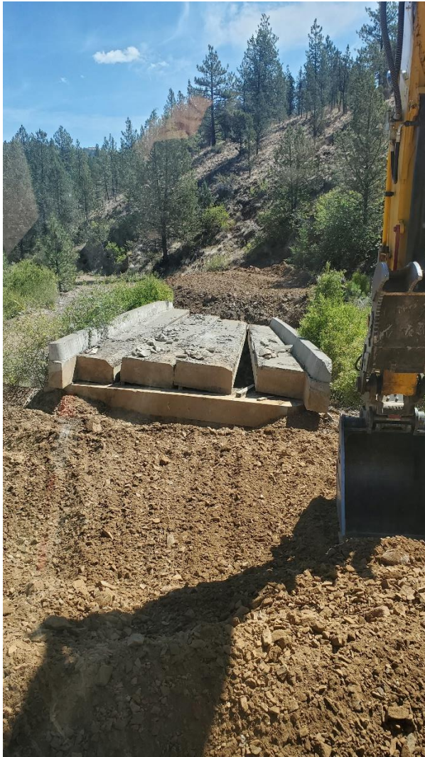
Left Photo - Exposing the Lower Foley bridge for transport to Dutchman Creek – August 8, 2023
