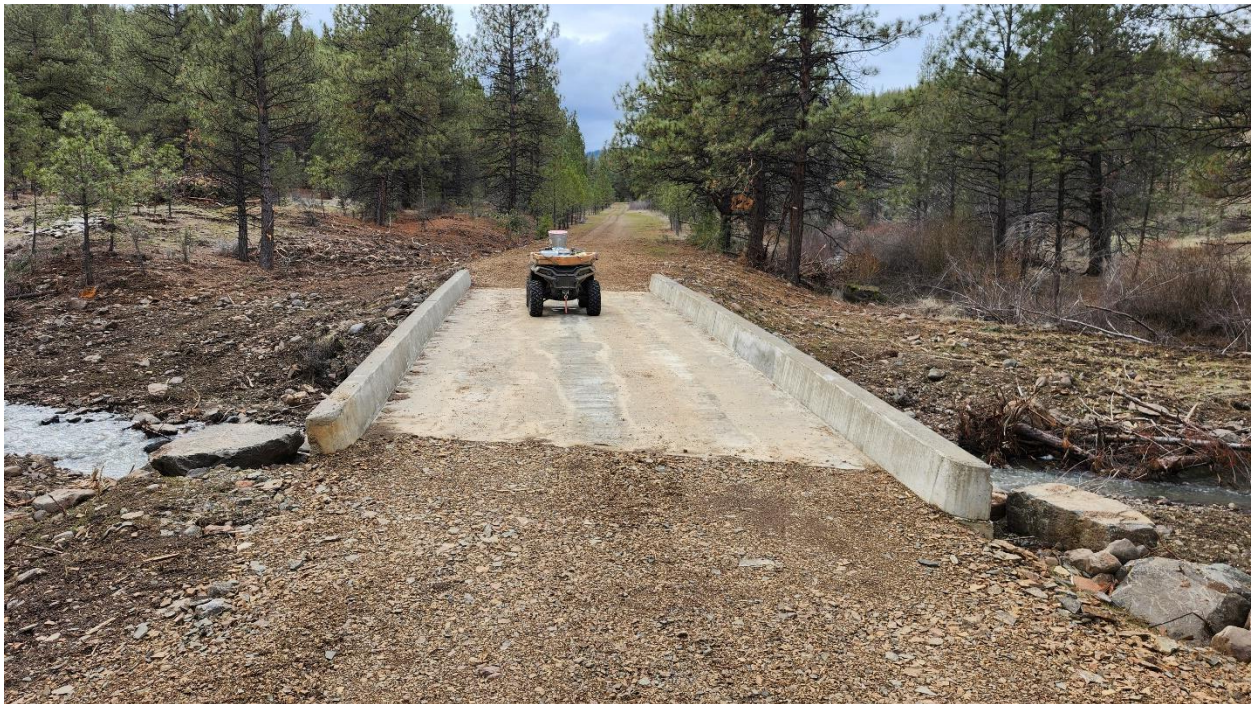
Completed Bridge, stream and floodplain work with water flowing – February 2, 2024
