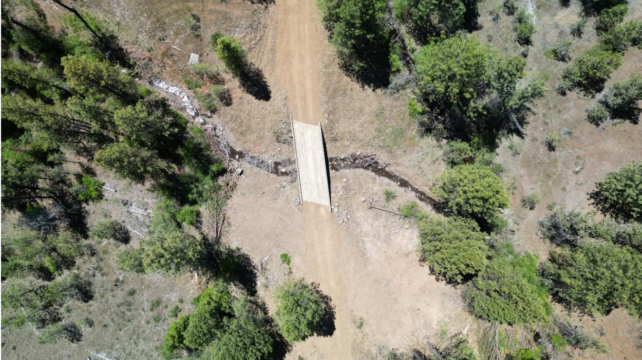
Aerial view of Dutchman Bridge – June 12, 2024
